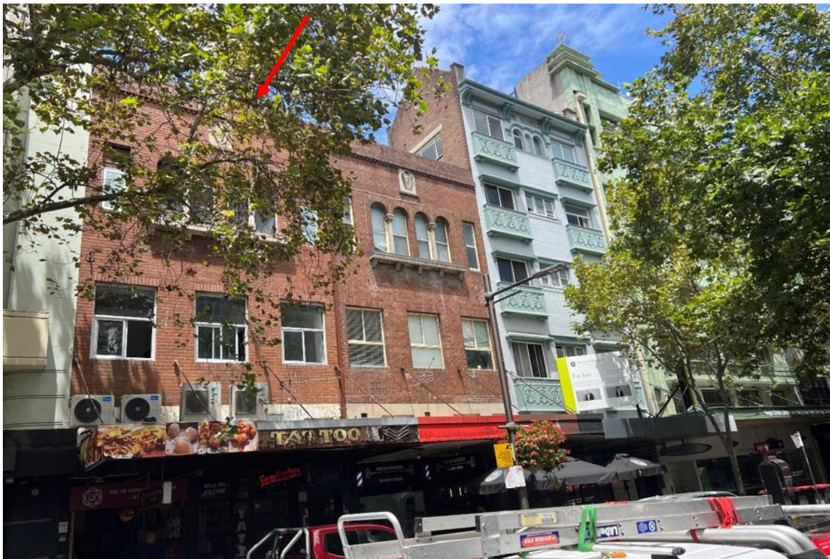
Figure 4: Neighbouring site at 40-44B Darlinghurst Road, including a mixed use building with ground floor retail and a licensed small bar
