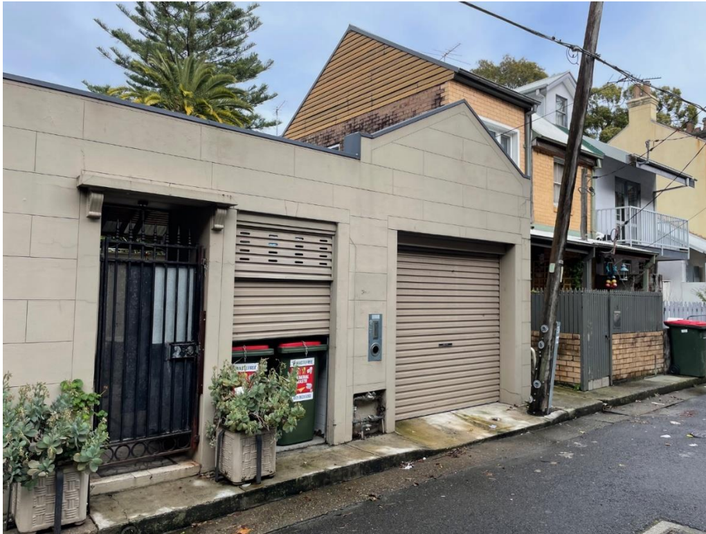
Figure 2: Site viewed from Wells Street
